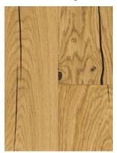
filled cracks with black putty (A)
